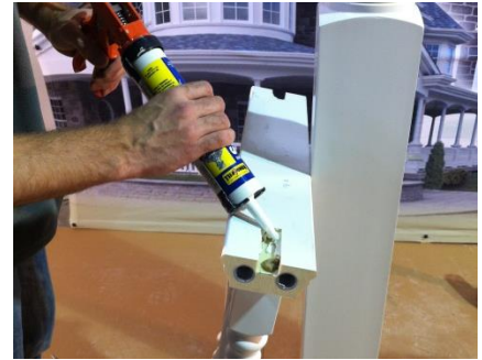
21. Apply a line of silicone caulking to the underside of each end of the top and bottom rail, where the plugs will be installed.
