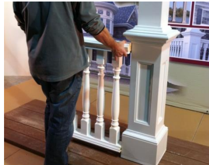
23. Position the rail in place
