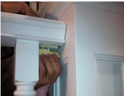
25. Install plugs to each end of the top and bottom rail.
