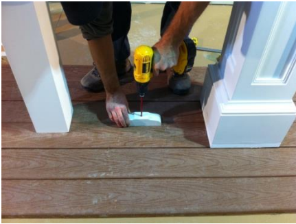
19. Fasten the support block with a screw. Make sure it is centered between each posts, or wall and post.
