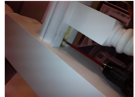
24. Fasten both ends of the top rail brackets with the supplied screws.
